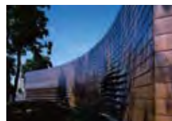
Cultural Center, Chateau-Rouge, Annemasse, F Cabinet R. Plottier, Lyon Ets. Fourquet, Perouges TECU® Classic
