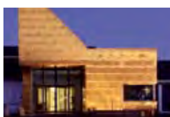
Haus Metzner, Residential and Care Centre for the Aged, Cremlingen-Gardessen, D Jörg Baumeister, m3xh, Braunschweig Musche GmbH, Magdeburg TECU® Gold
