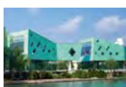
Yefei's Creative Street, Shanghai Will Alsop Architects, London, GB; U/Jiang Architects & Engineers, Shanghai Hanchang Industrial Development Co., Shanghai TECU® Patina, TECU® Oxid, TECU® Bronze
