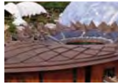
THE CORE, Information Centre for the Eden Project, Cornwall, GB Nicholas Grimshaw & Partners, London Richardson Roofing Co. Ltd., Staines TECU® Classic
