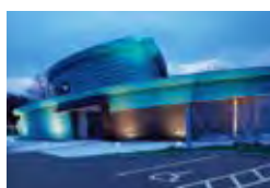
Maggie's Highlands Cancer Caring Centre at Raigmore Hospital, Inverness, GB Page & Park Architects, Glasgow W B Watson Ltd., Stewarton TECU® Patina, TECU® Oxid
